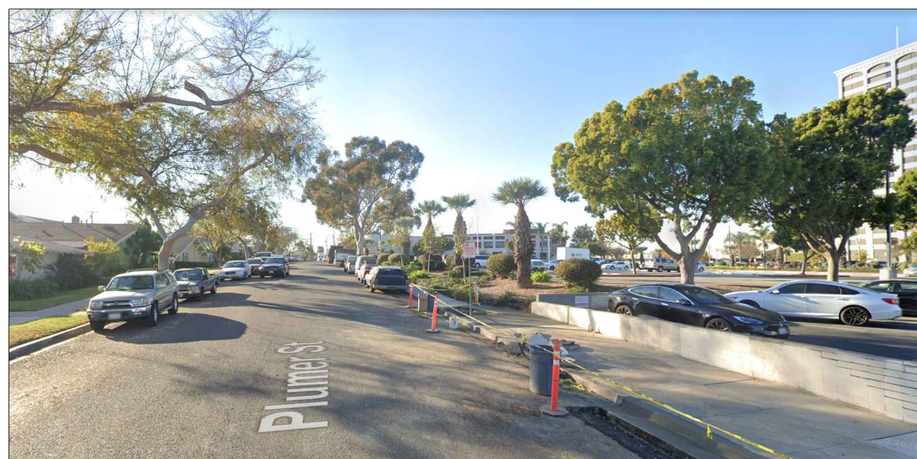
VIEW LOOKING WEST FROM PLUMER ST. 008
