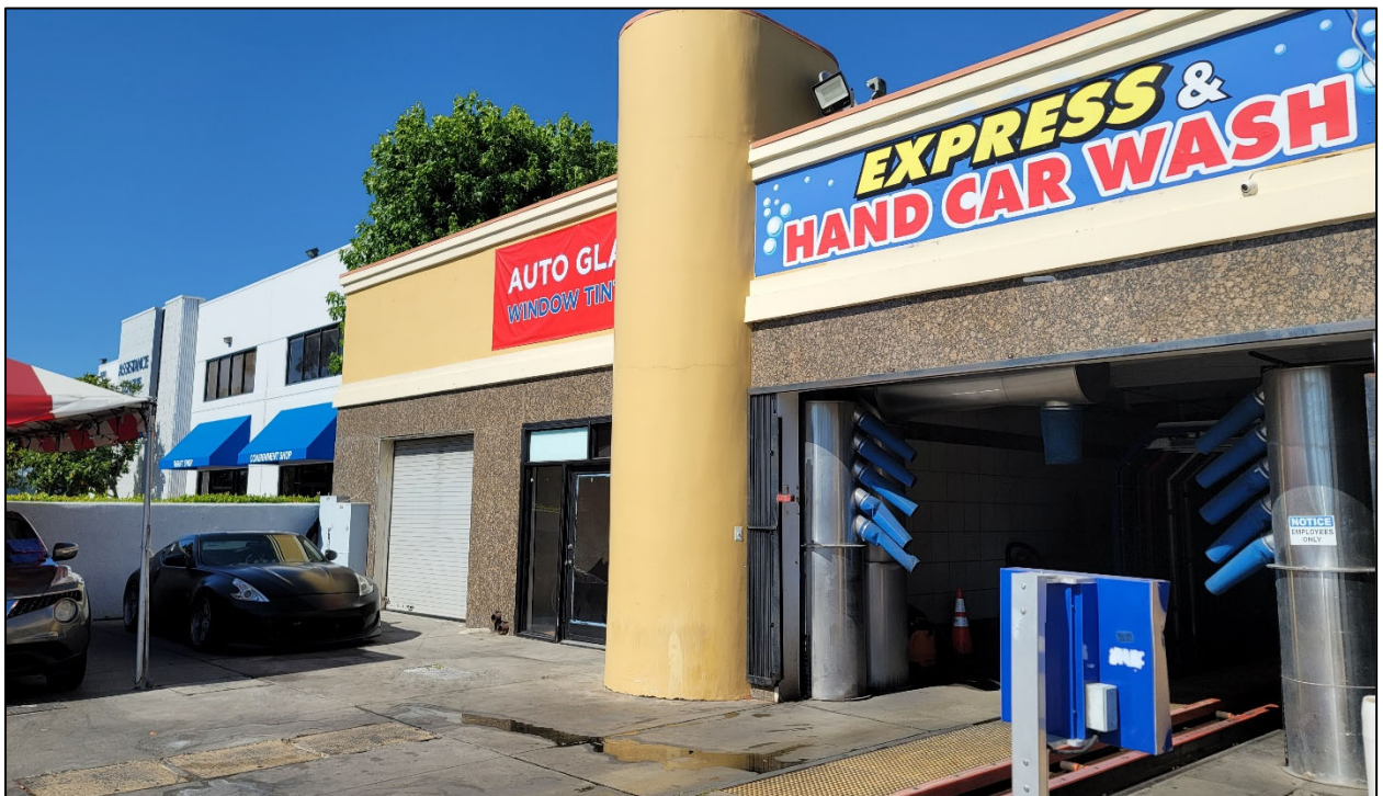
View of the existing facility from the side of the property facing Fairview Road.
