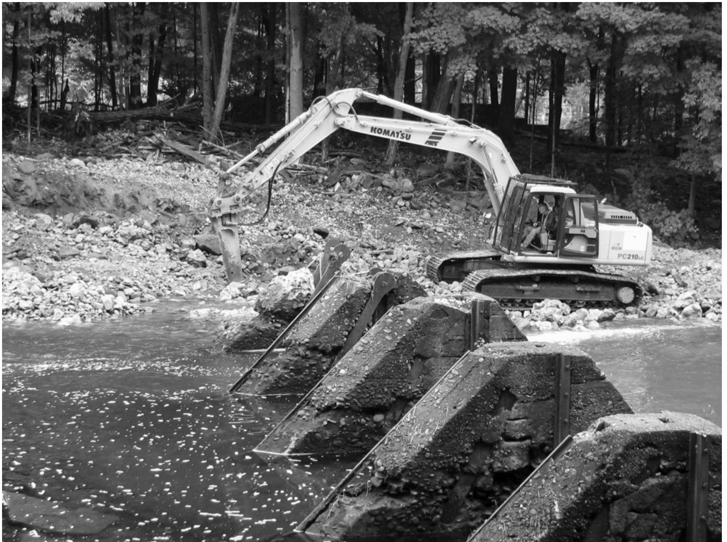
CUDDEBACKVILLE DAM, NEW YORK Start of breach during demolition of the Cuddebackville dam on the Neversink River at Cuddebackville, New York in September, 2004. © George Schuler/TNC
