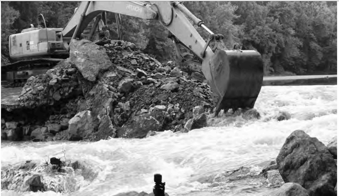
ROARING RIVER DAM DIGGING OUT A power shovel tears away the old deteriorating dam on Tennessee's Roaring River. © Paul Kingsbury/The Nature Conservancy
