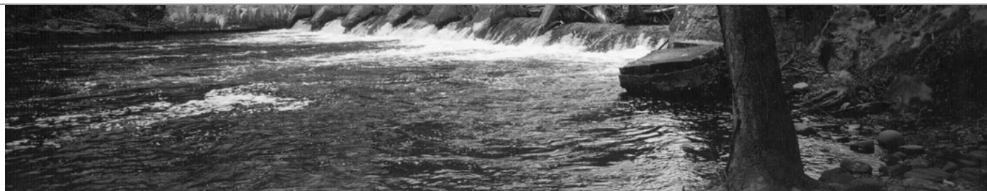
CUDDEBACKVILLE DAM Photo of the dam prior to its 2004 demolition on the Neversink River at Cuddebackville, New York. © Mark Godfrey/TNC
