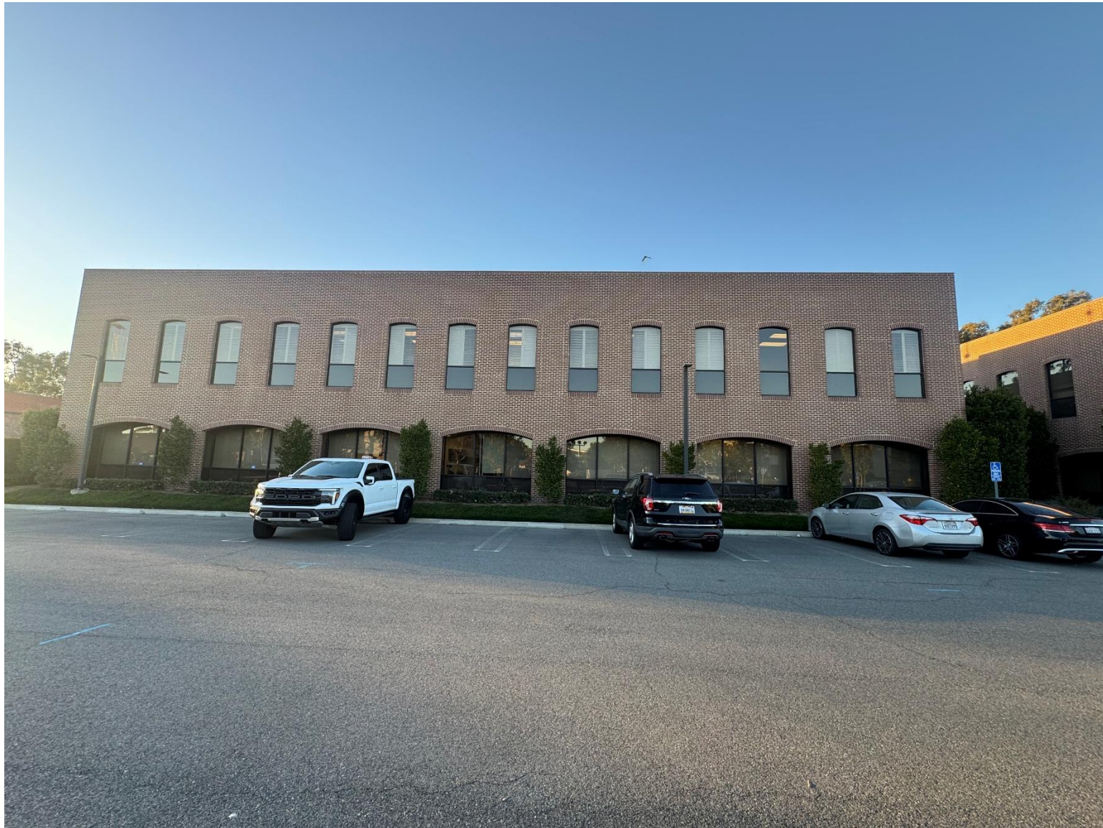
3146 Red Hill Ave (Rear View)
