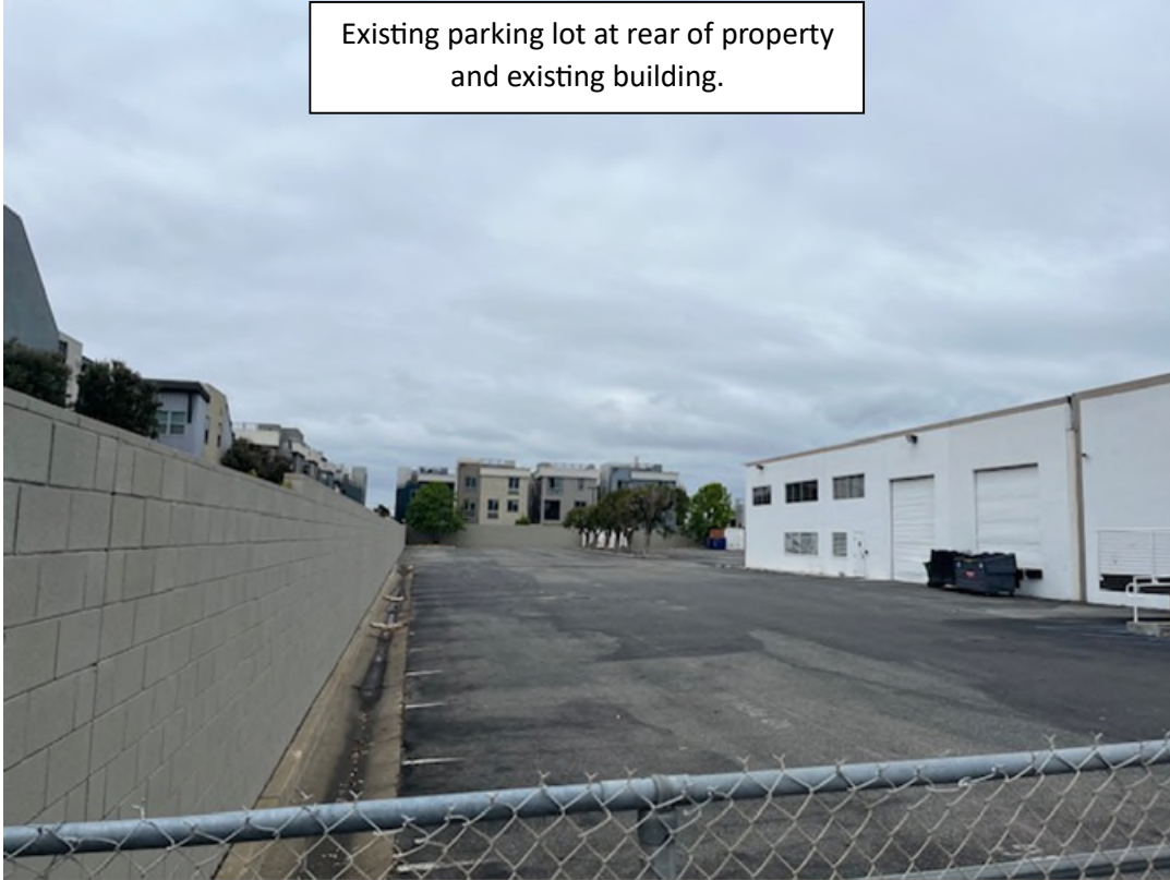
Existing building to be demolished.
