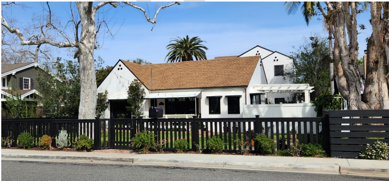
Figure 1: 208 Magnolia Street, view looking north. Source: GPA Consulting, February 2023.
