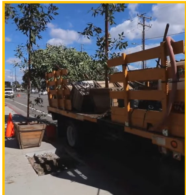
NEW TREES ALONG PLACENTIA AVENUE
