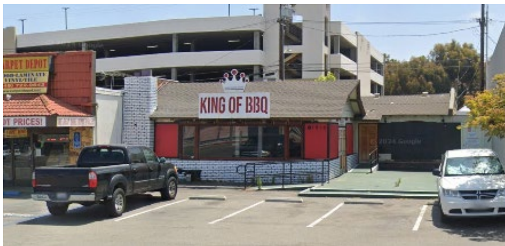
Image 1 - Existing Condition, 1912 Harbor Boulevard
