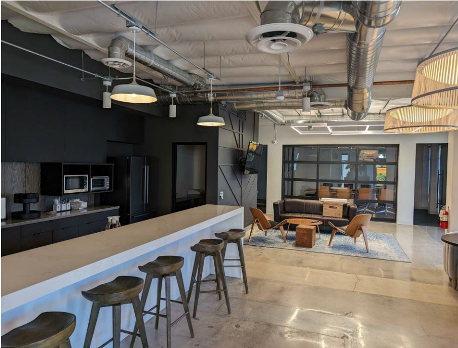
15. View of the interior of Unit D-101 showing non-asbestos sheetrock and joint compound.
