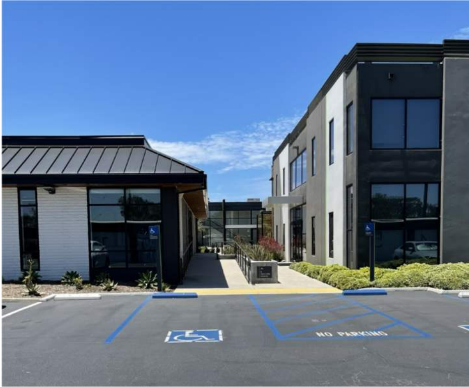
Image 7 - Breezeway Between Bldg. C&D Looking West
