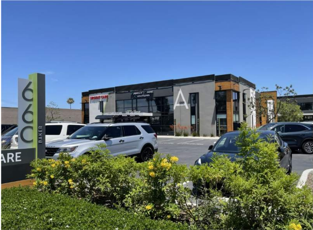
Image 1 - South Side of Building A
