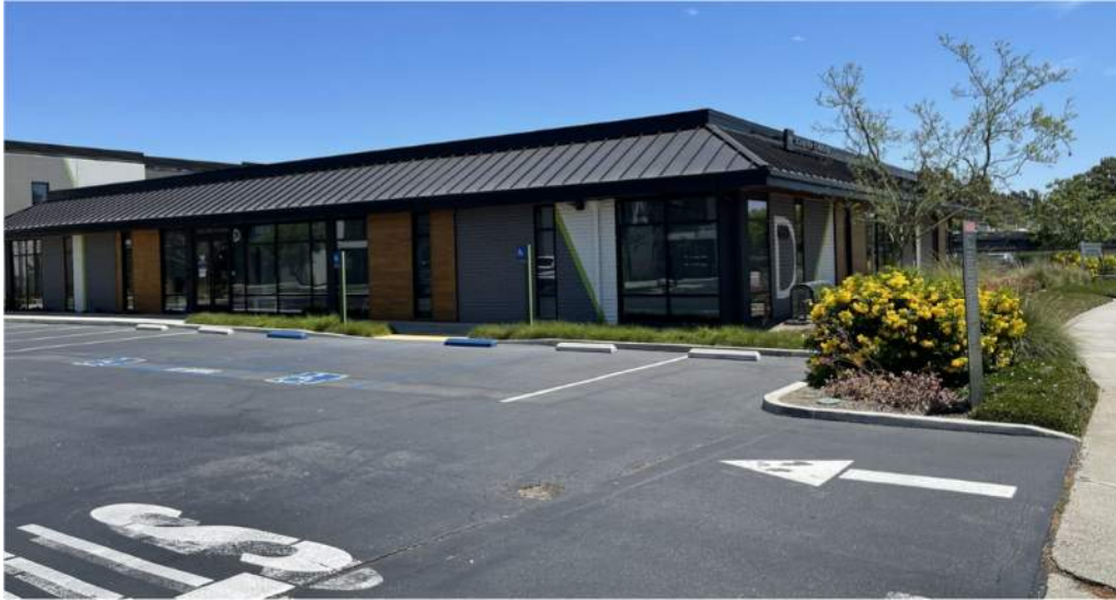
Image 3 - South-West corner of Building D
