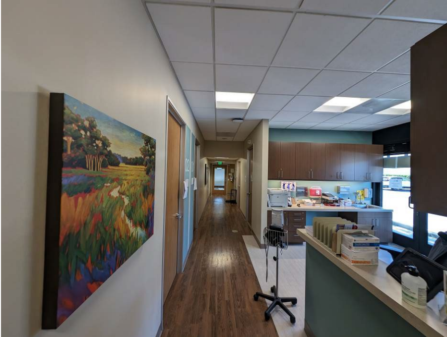
19. View of the interior of Unit A-101 showing non-asbestos sheetrock, joint compound, and ceiling tile.
