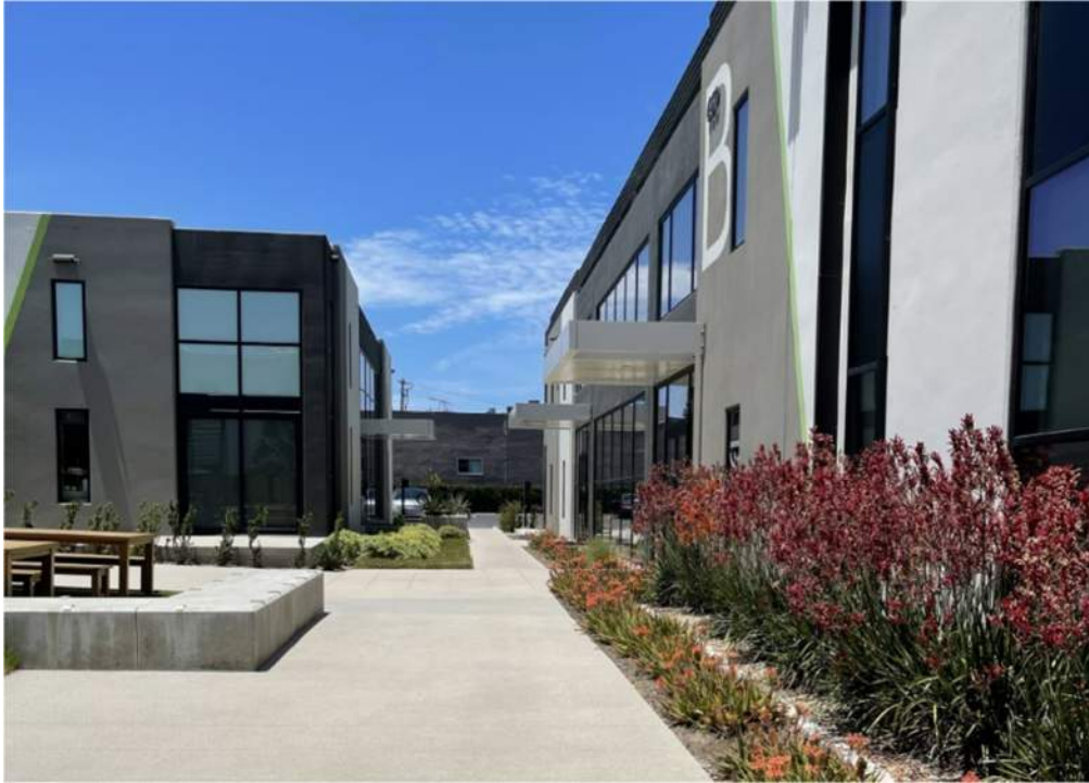
Image 5 - Breezeway Between Bldg. A&B Looking West
