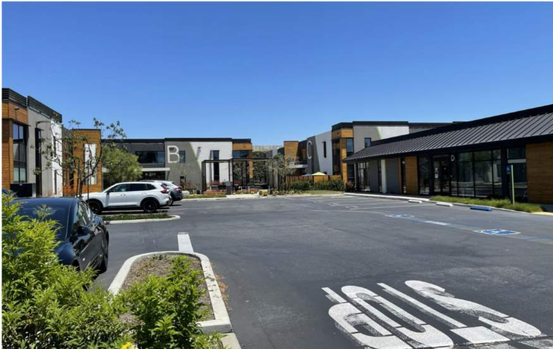
Image 2 - South Side of Buildings B, C, & D
