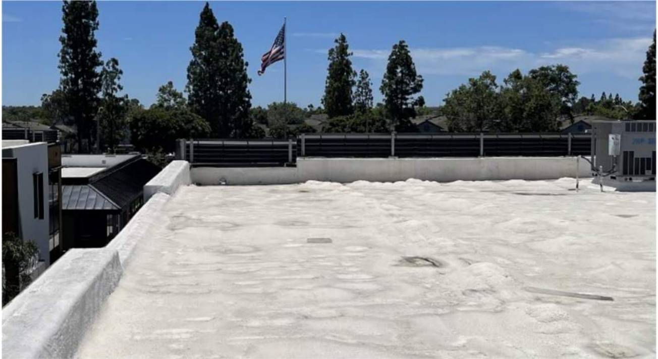
Image 12 - Typical Roof Slope to Corner Drain and Scupper
