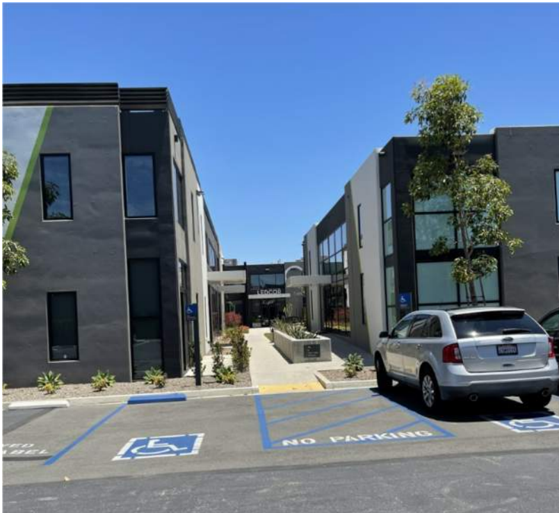
Image 10 - Breezeway Between Bldg. A&B Looking East
