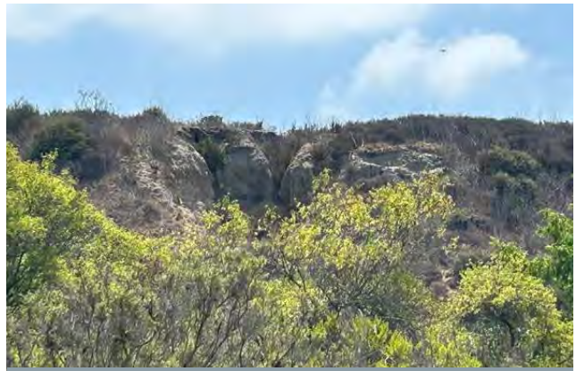
Eroded Slope at Fairview Park Project Site
