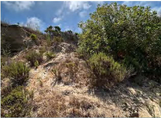
Eroded Bluff at Fairview Park Project Site
