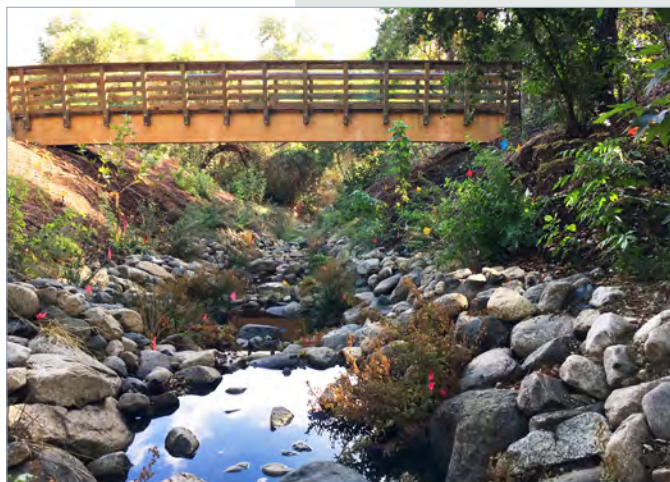
New Pedestrian Bridge over Rehabilitated Berkshire Creek
