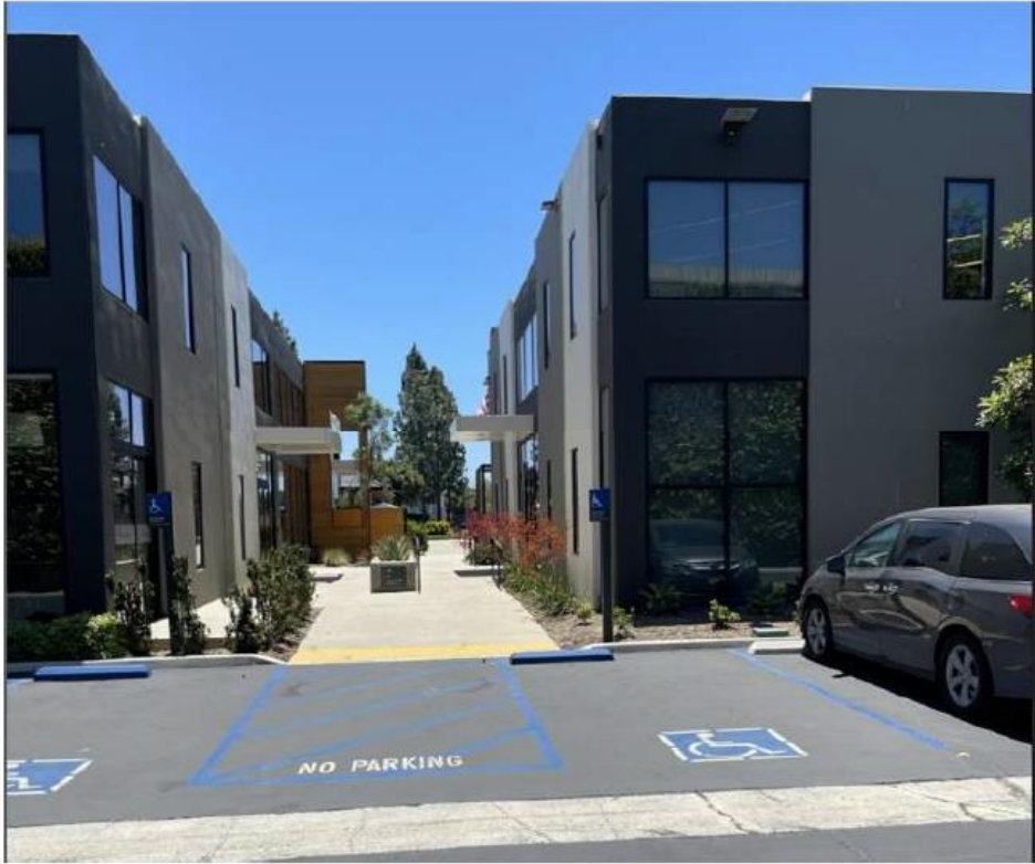
Image 9 - Breezeway Between Bldg. B&C Looking South
