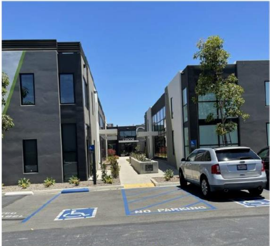
Image 10 - Breezeway Between Bldg. A&B Looking East
