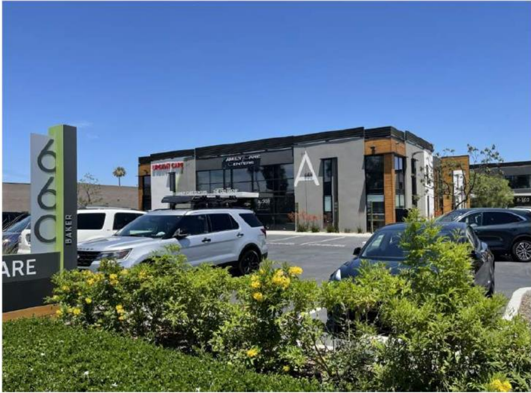
Image 1 - South Side of Building A
