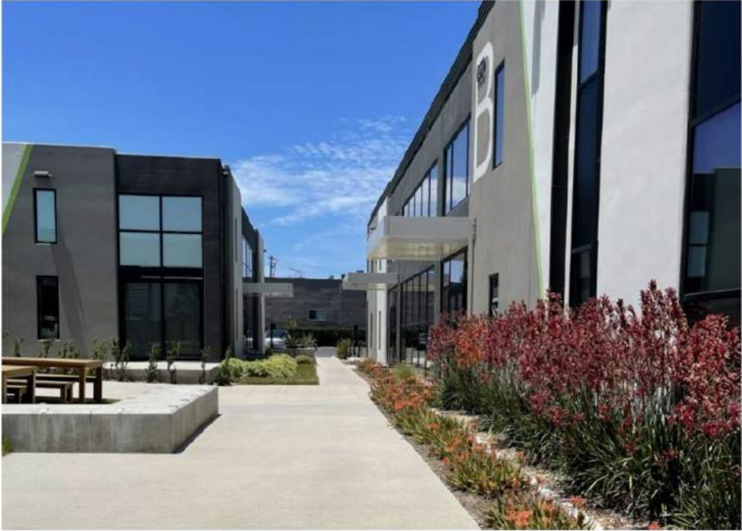
Image 5 - Breezeway Between Bldg. A&B Looking West
