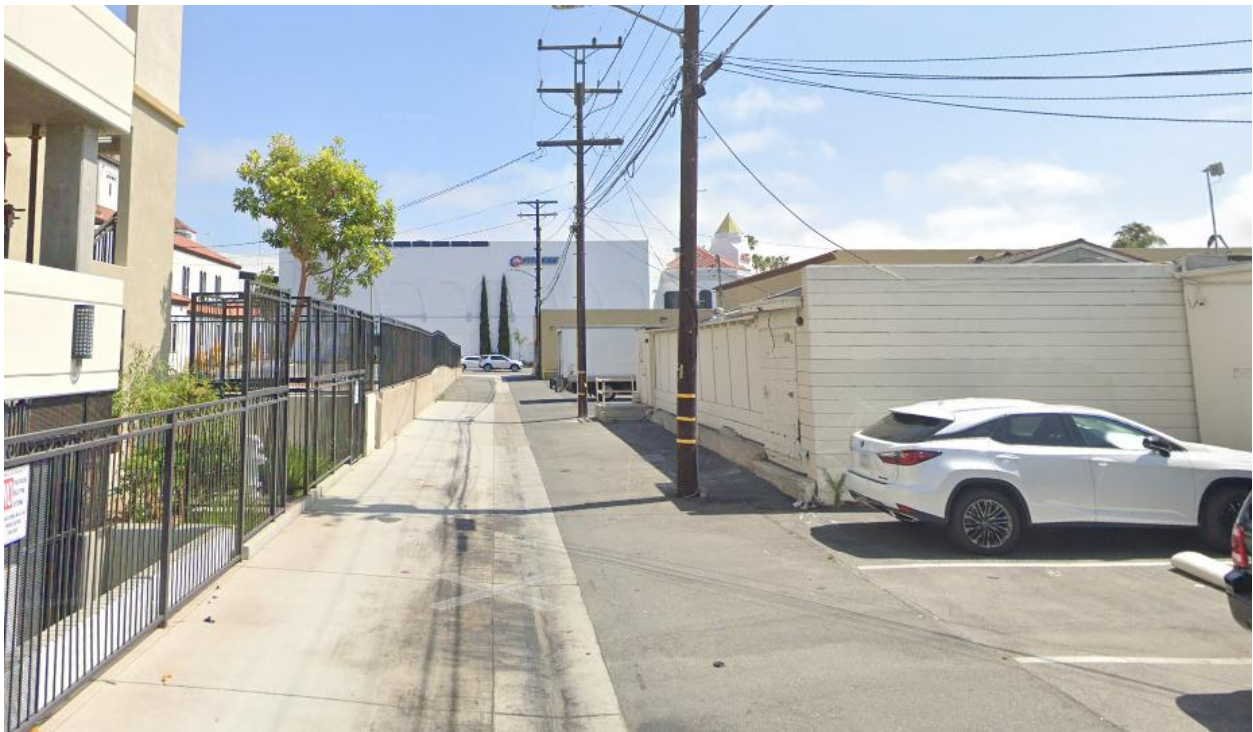
View of the existing building (right) from the alley. Photo facing south toward Triangle Square.
