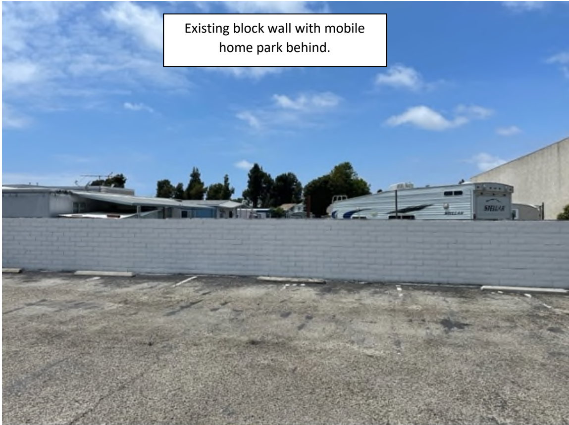
Existing trash enclosure.
