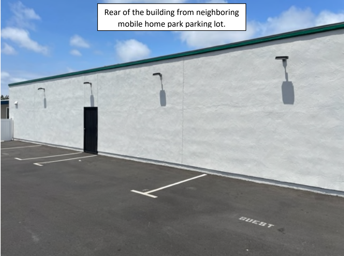
Front block wall to be removed
