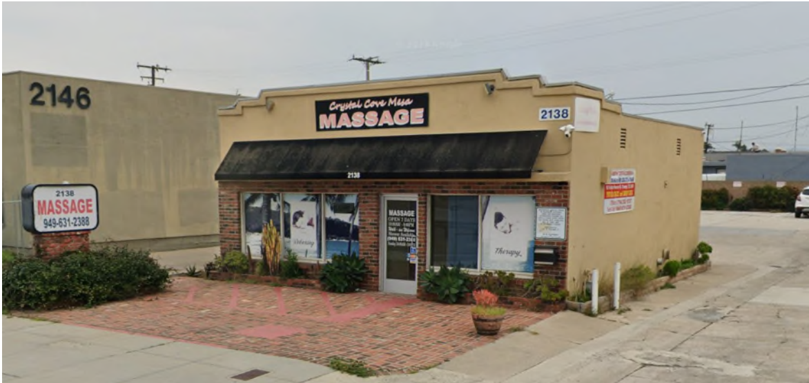
Image 1 – Existing Condition, 2138 Newport Boulevard
