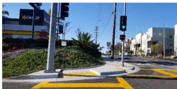
Newport Boulevard and Industrial Way
