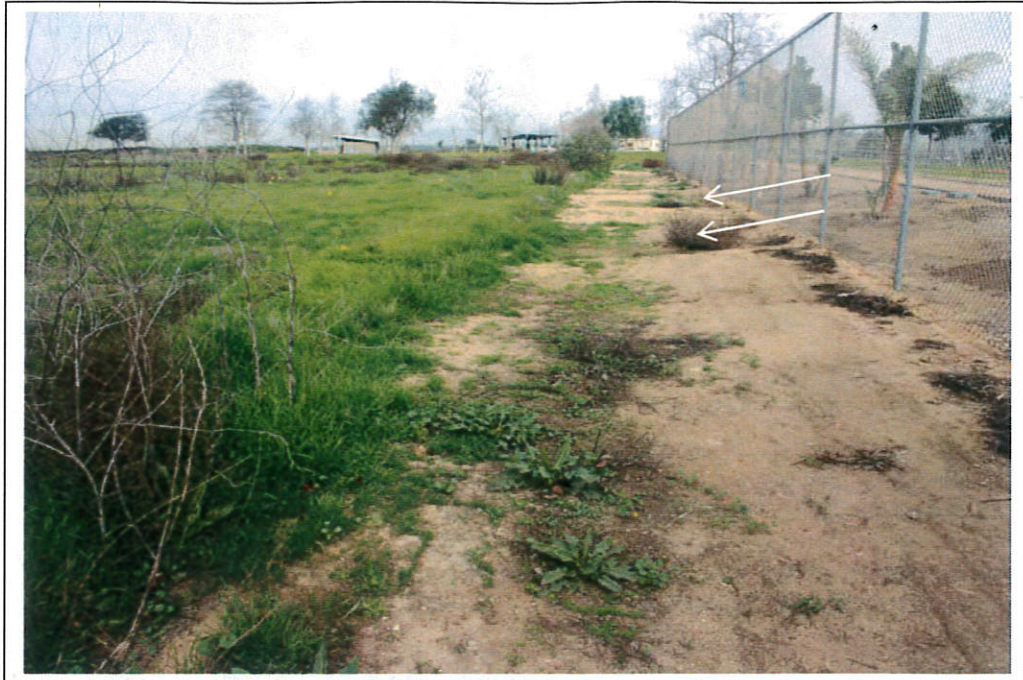
Photograph 1: View of foot path facing north. Note arrows pointing to depressions which will be smoothed to ensure positive drainage to Vernal Pools 5 and 6. The restored foot path will be re-vegetated with native upland species. Vernal Pool 5 is located in the top left of photo, and Vernal Pool 6 is located in the bottom left.
