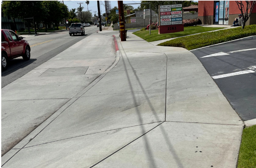
Driveway ramp that hampers pedestrian using sidewalk
