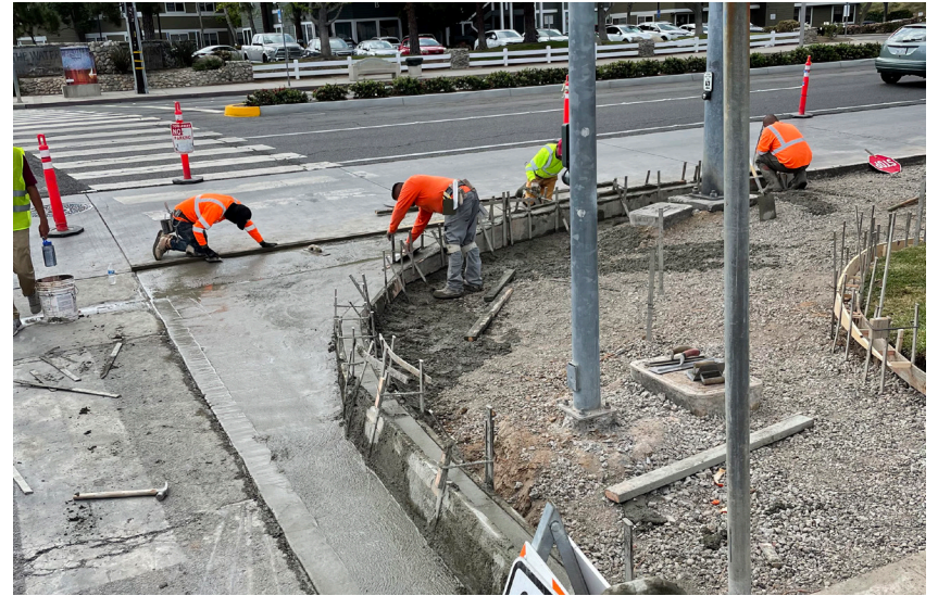
Construction workers installing new curb ramp
