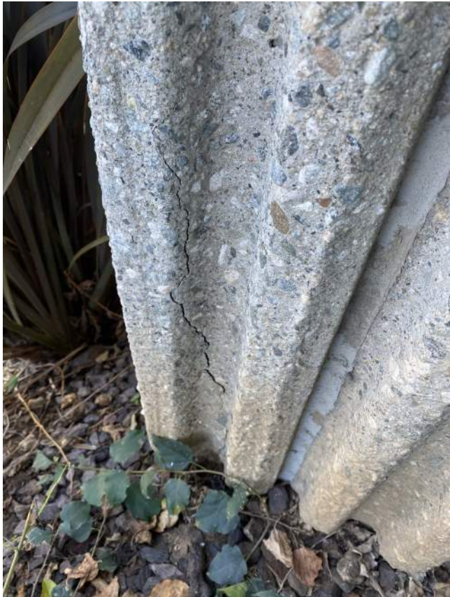
FIG 11: MINOR CRACKING / SPAWLING IN EXISTING TILT-UP WALL
