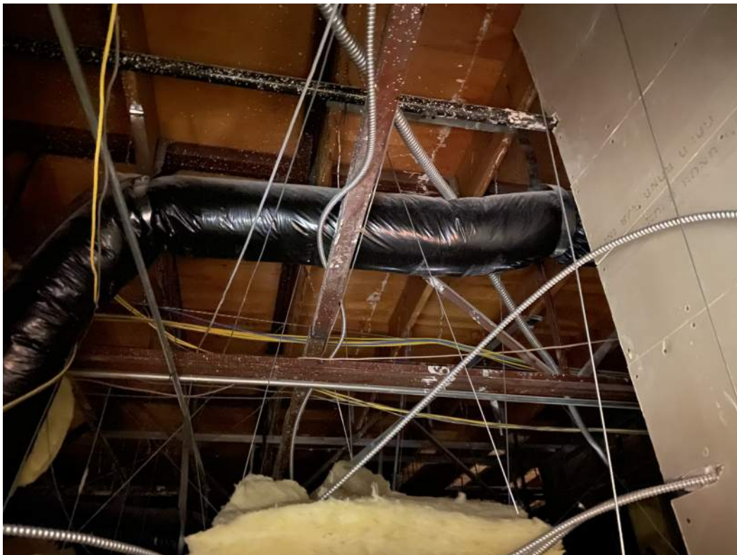
FIG 6: TYPICAL FLOOR STRUCTURE - 2x10 JOISTS, OWSJ, OWSJ GIRDER
