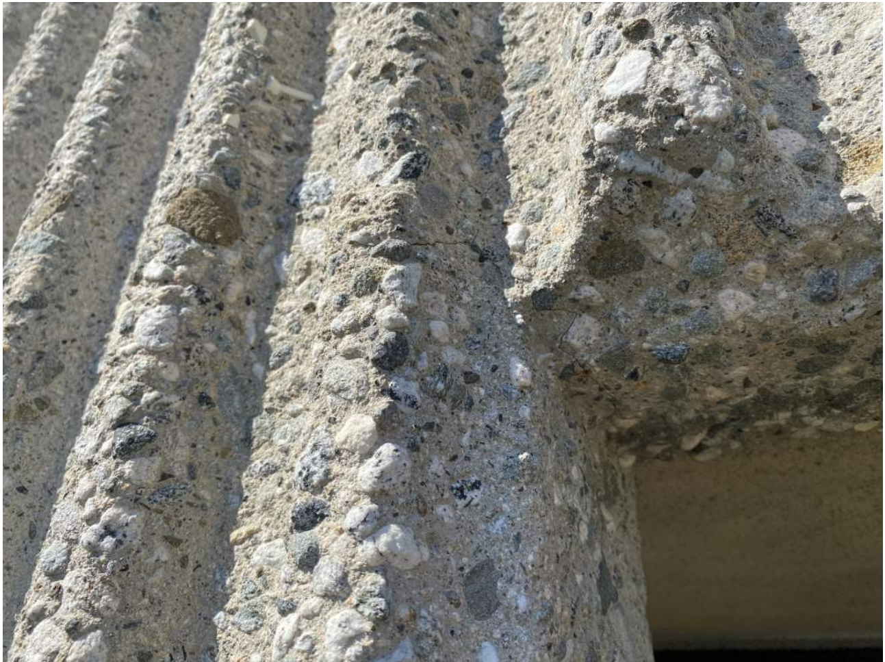
FIG 12: MINOR CRACKING IN CONCRETE TILT-UP LINTEL TO WALL
