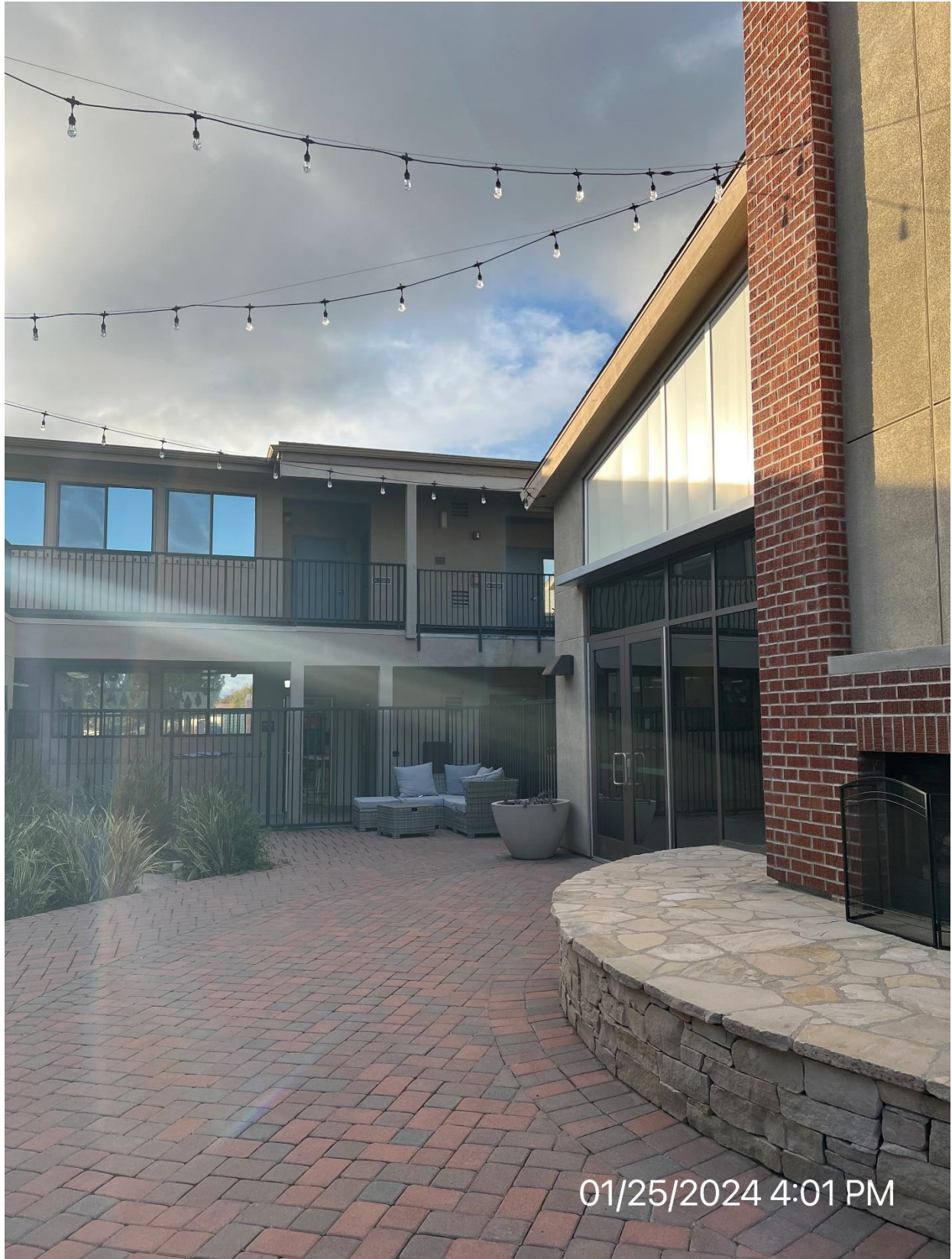
Photo 3 – Fireside & Classroom Buildings
