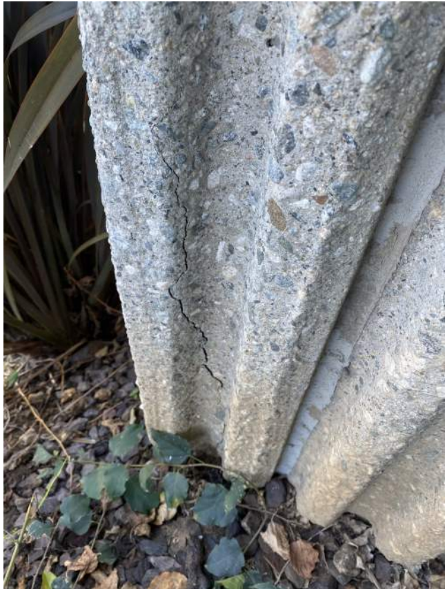
FIG 11: MINOR CRACKING / SPAWLING IN EXISTING TILT-UP WALL
