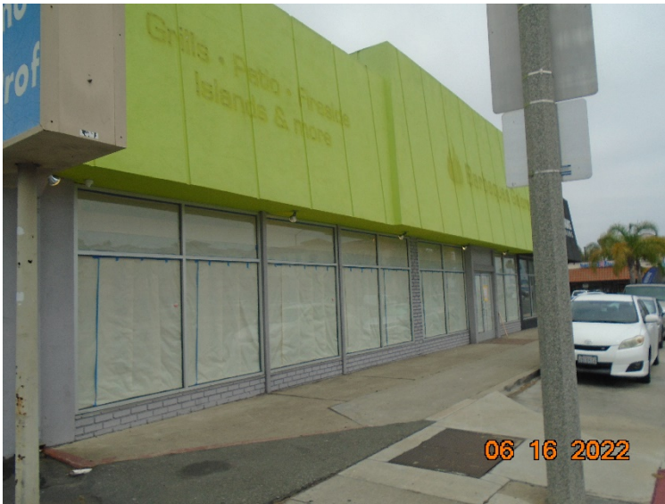
Existing building front façade facing Harbor Blvd. to be updated with new façade, paint, and signage
