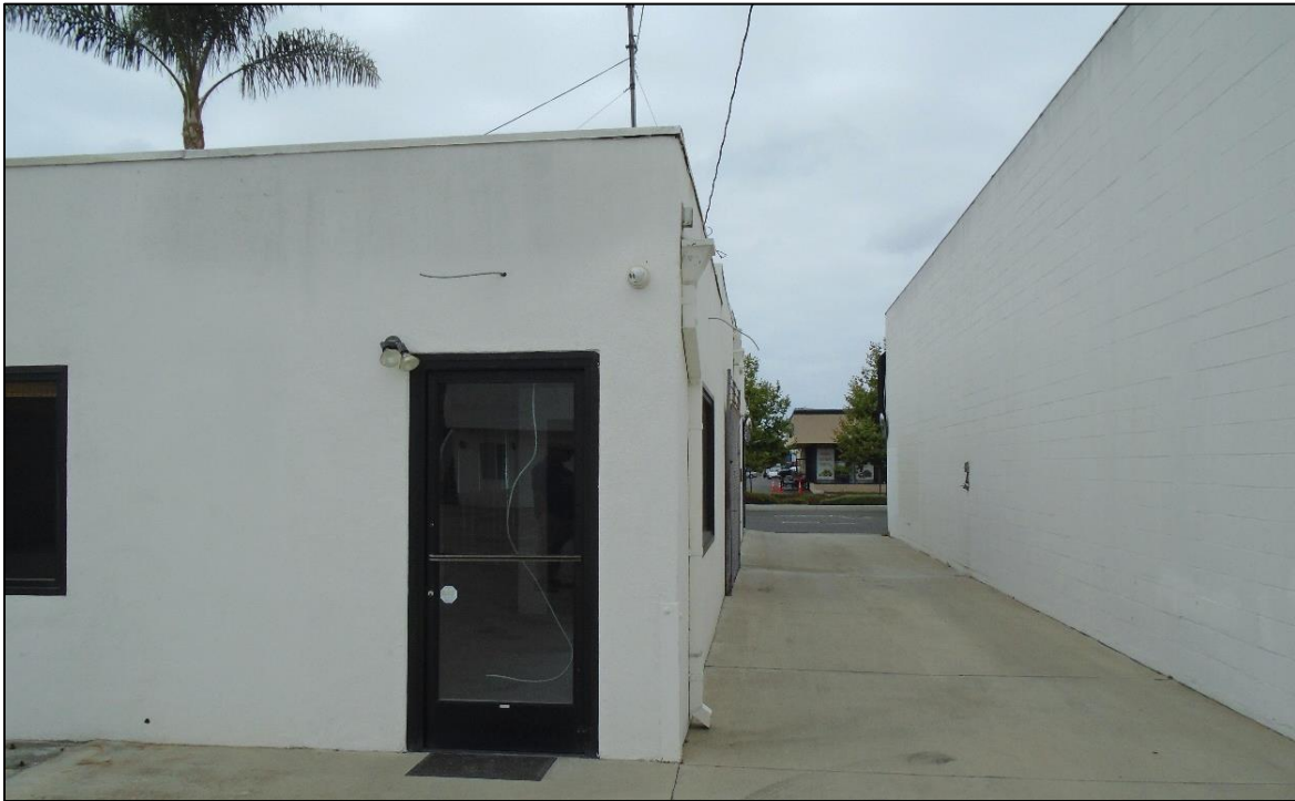
View of the front building and driveway looking toward Harbor Boulevard
