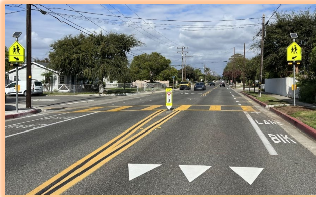
Rectangular Rapid Flashing Beacon at Santa Ana Avenue and Esther Street
