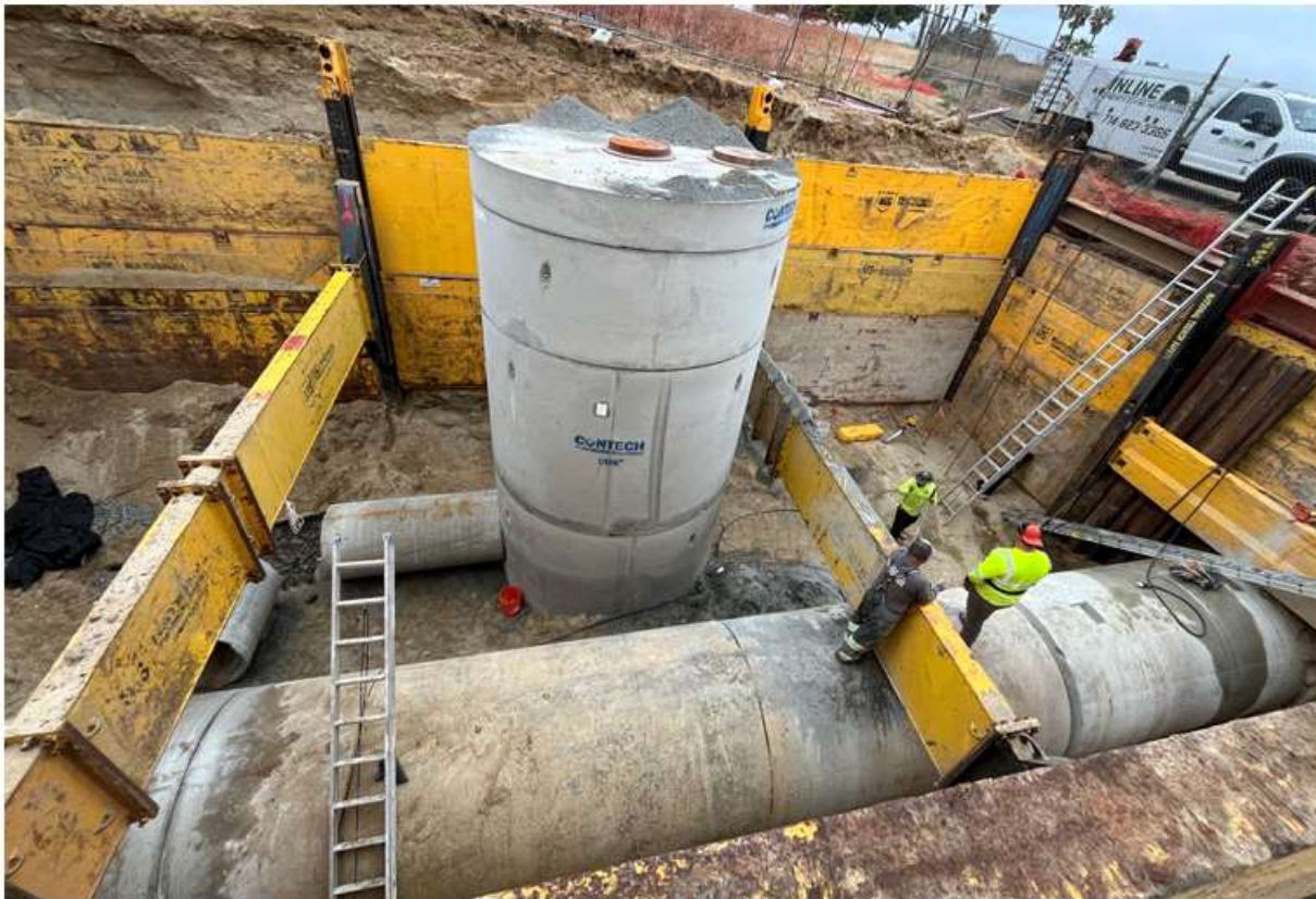
Newly installed Hydrodynamic Separator Unit
