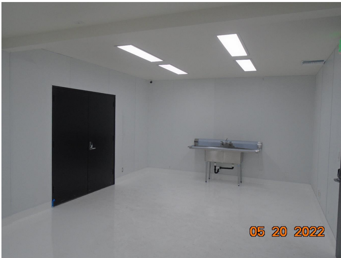
PA-22-13 Site Photos 3505 Cadillac Avenue, Unit F3
