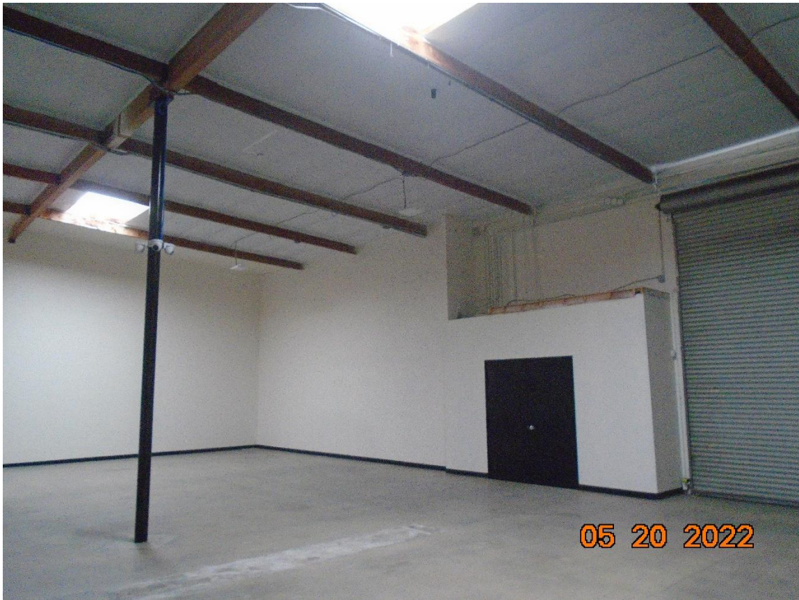
PA-22-13 Site Photos 3505 Cadillac Avenue, Unit F3
