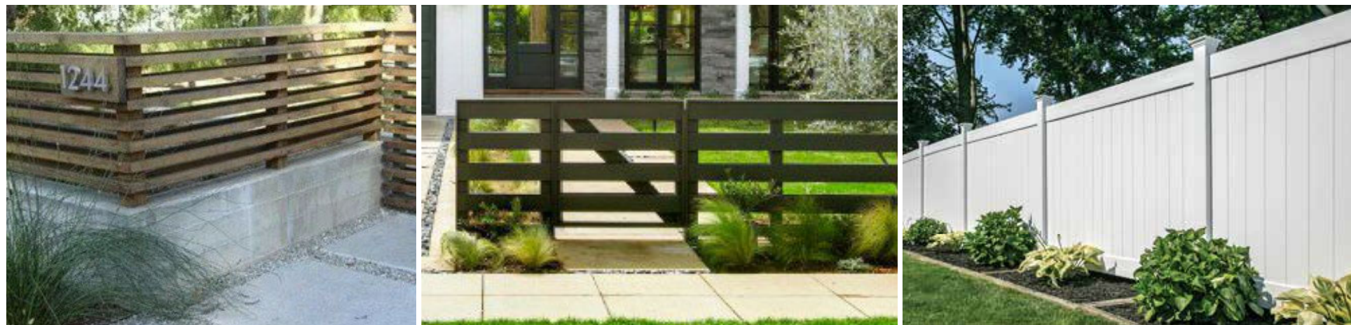
WOOD SLAT FENCE ON LOW CONCRETE WALL - MAX HT 30" 6-0" VINYL PRIVACY FENCE
