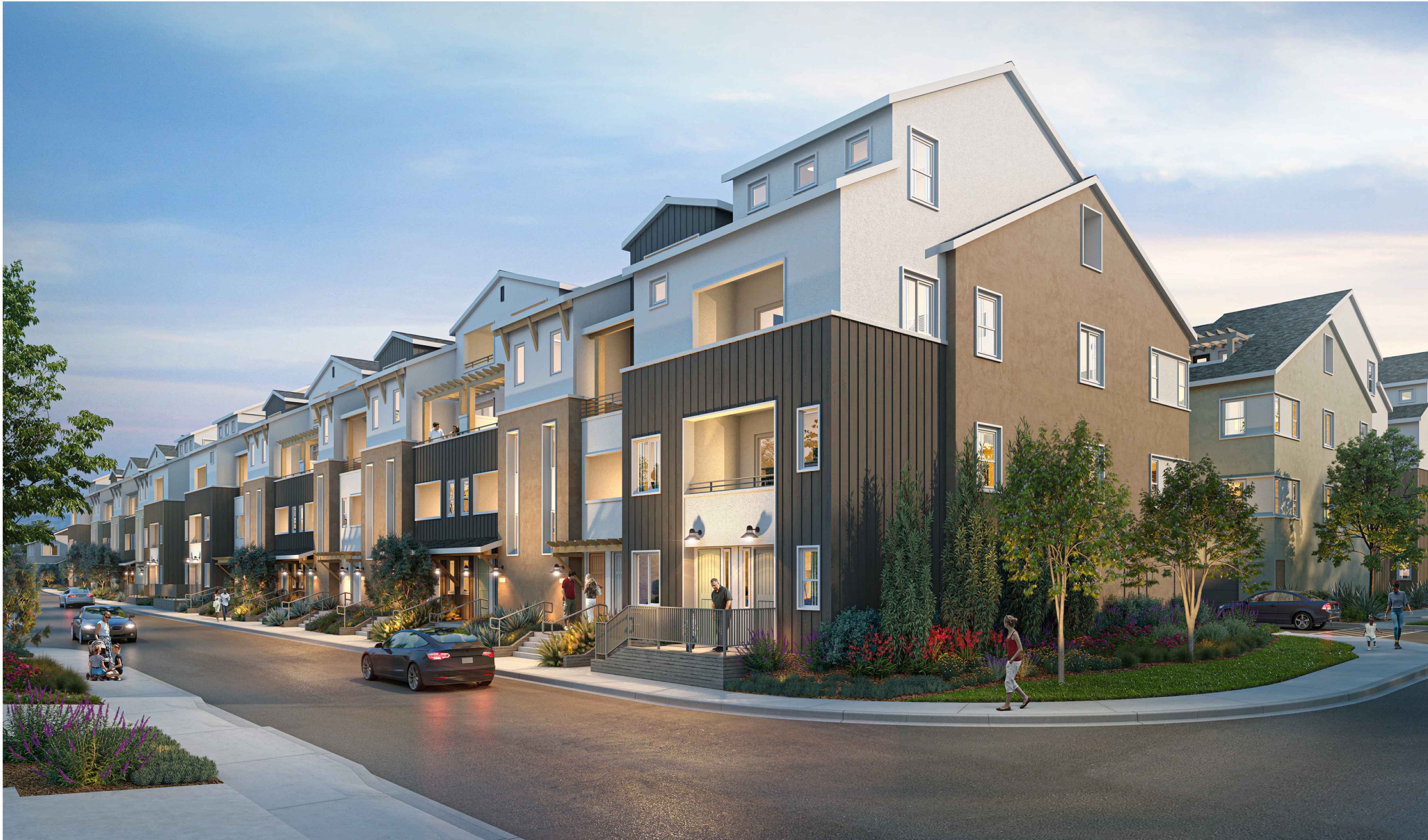
VIEW OF STACKED FLATS DOWN PRIVATE DRIVE D
