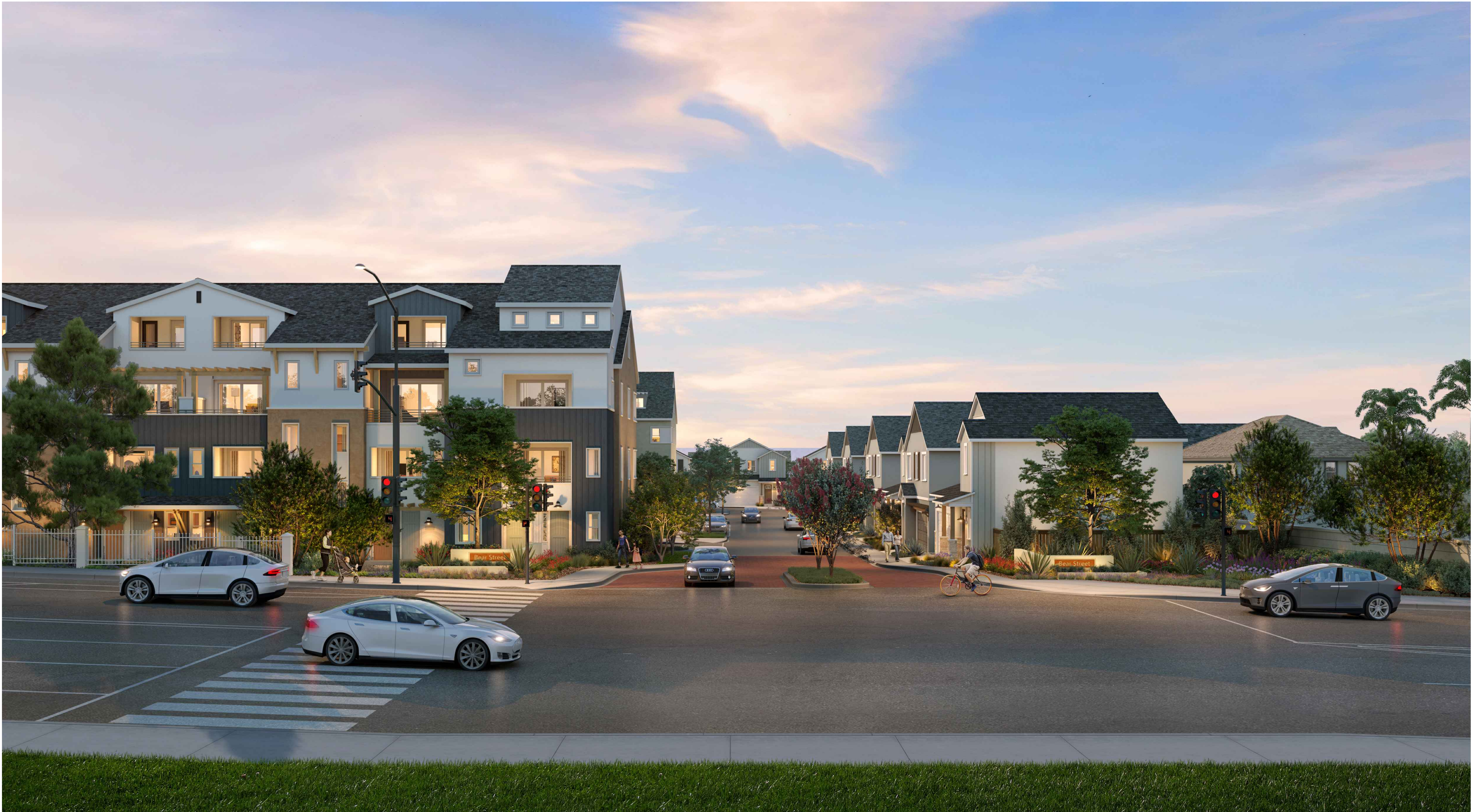
VIEW OF PROJECT ENTRY
