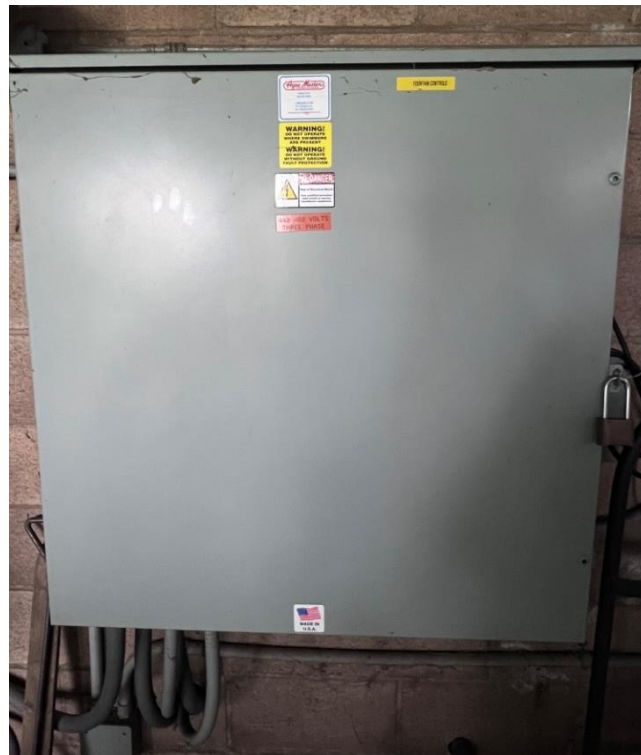
Figure 2-14: Floating Fountain Control Panel
