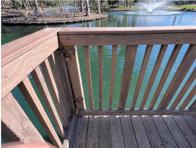
Figure 2-2: Maintenance Boat Dock at Pier Deck with Lockable Gate
