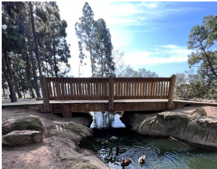
Figure 2-5: Wooden Bridge at Pond 1
