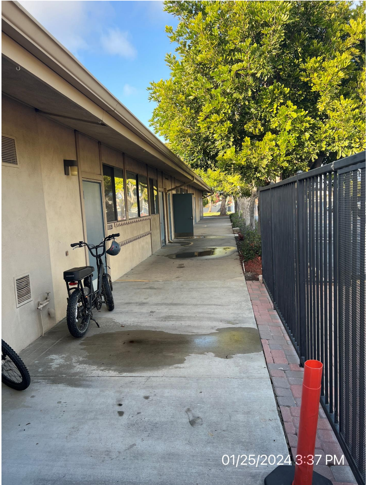
Photo 2 – Eastern Elevation of Gym Building
