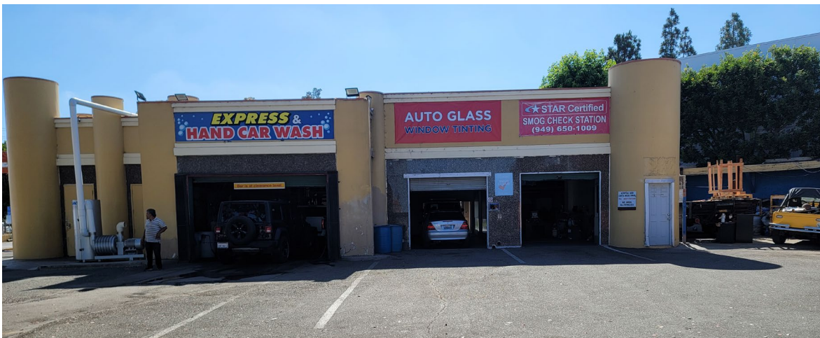
Image 1 – 2285 Newport Boulevard as Viewed Facing West
