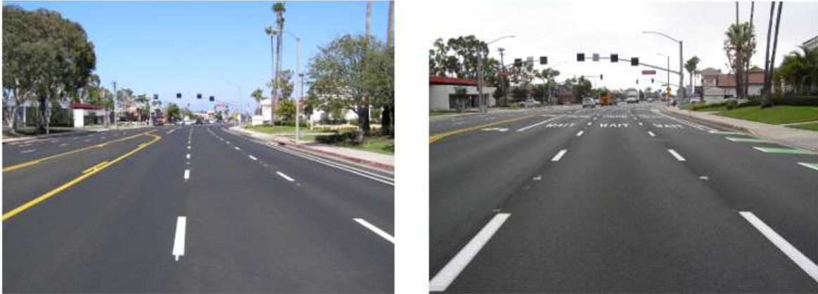
Adams Avenue (After Construction)
