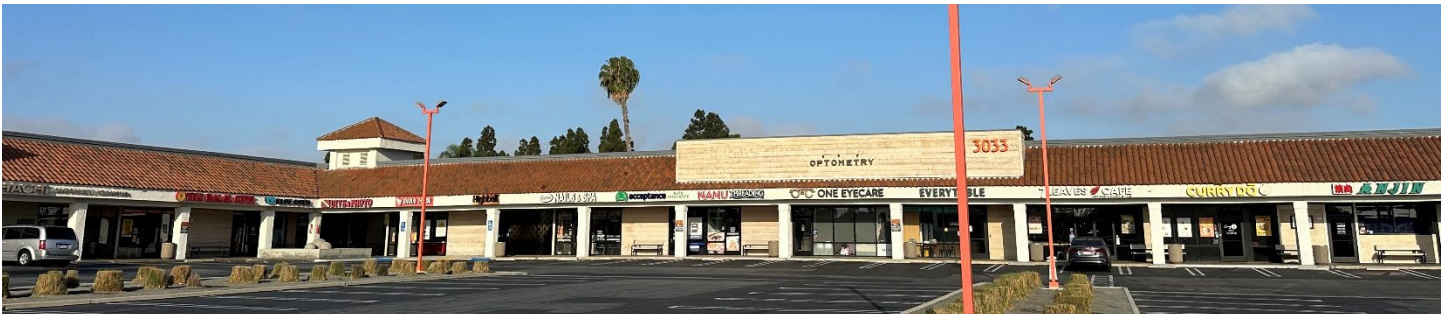
2. Portion of existing multi-tenant building - facing Bristol Street
