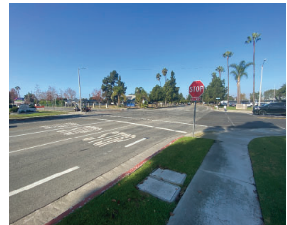
Multi-lane STOP controlled intersection on Baker Street
