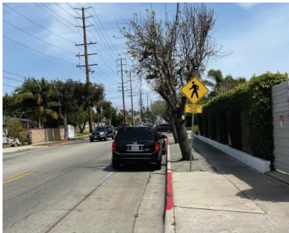
Pedestrian signage south of Harbor Blvd without mid-block marked crosswalks
