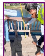
LOW RAILING SECTION AT PIER DECK
