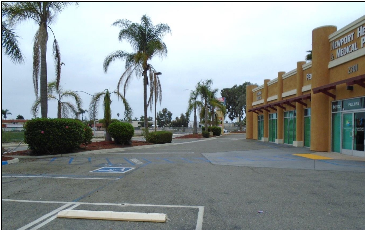
View from the middle of the parking lot (looking south)
