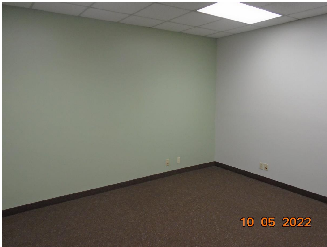
PA-22-27 Site Photos 3505 Cadillac Ave., Unit O-209A
