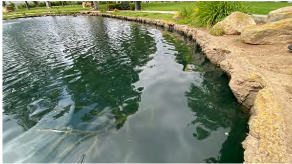
The existing shorelines and edges are damaged and at the End of their useful life, and lack of landscaping creates muddy condition.
