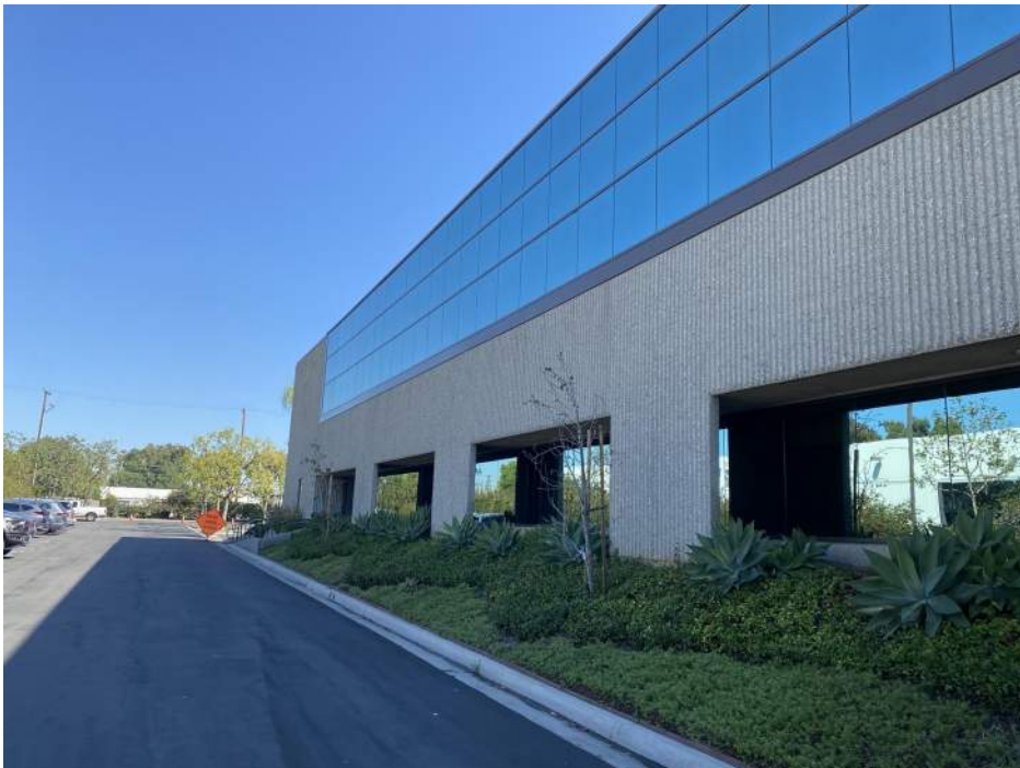
FIG 2: NORTHWEST ELEVATION OF BUILDING
