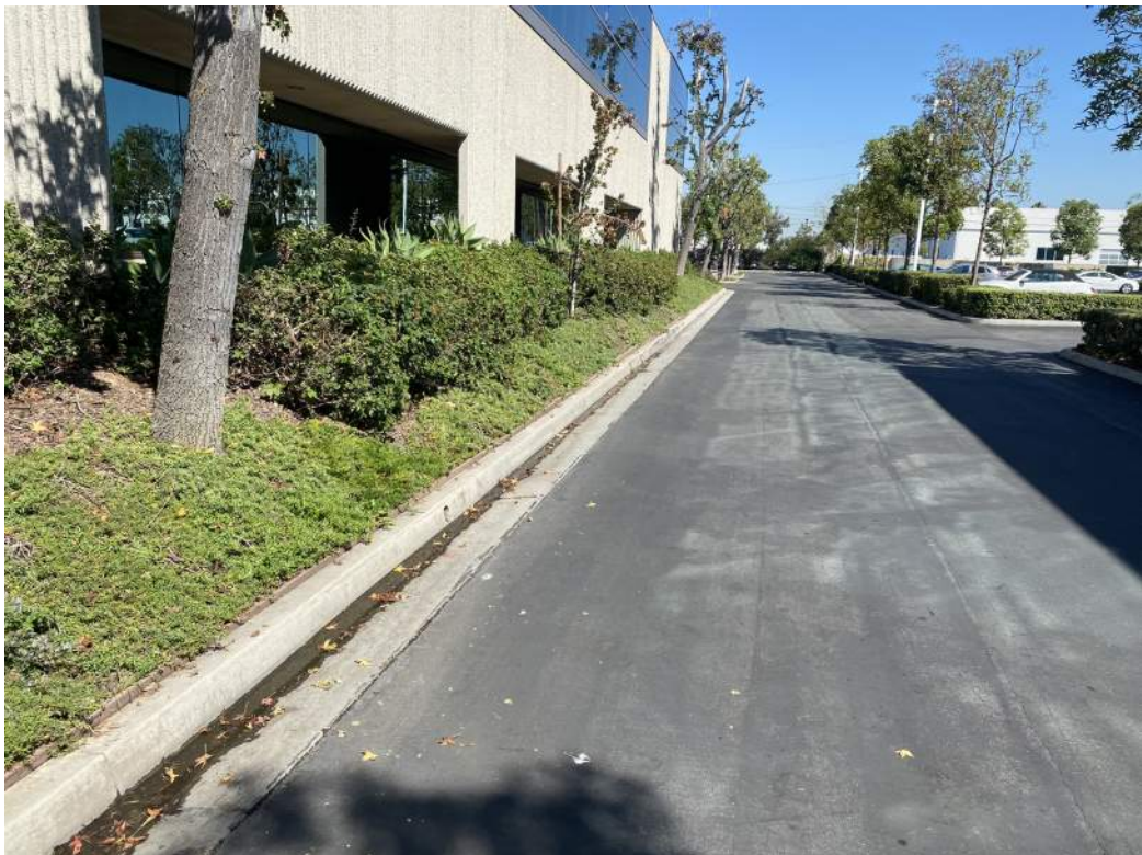
FIG 4: SOUTHEAST ELEVATION OF BUILDING WITH GUTTER
