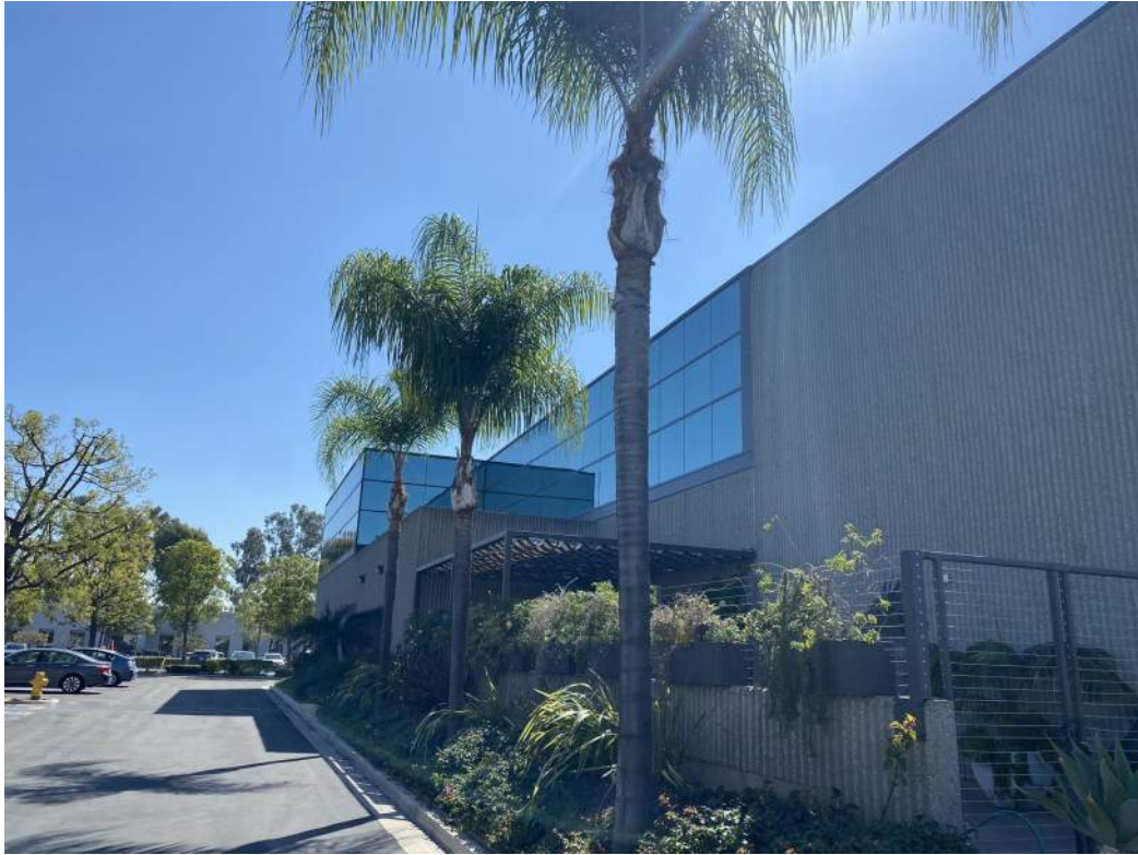
FIG 3: NORTHEAST ELEVATION OF BUILDING WITH EXTERIOR BACK PATIO
