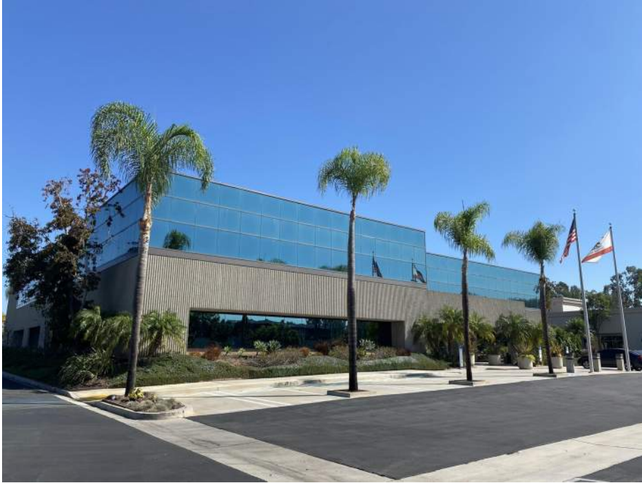
FIG 1: BUILDING EXTERIOR LOOKING FROM WEST
