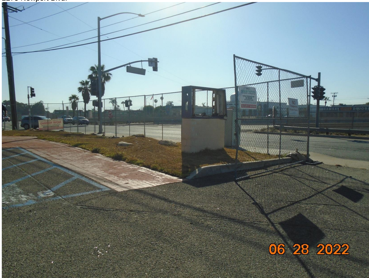
PA-21-24 Site Photos 2275 Newport Blvd.
