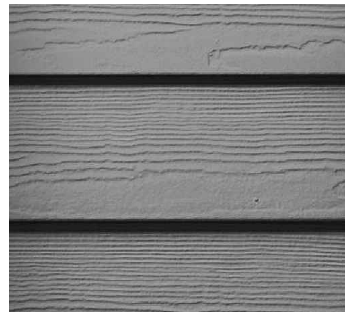
3 HORIZONTAL SYNTHETIC BOARD JAMES HARDIE OR SIMILAR
