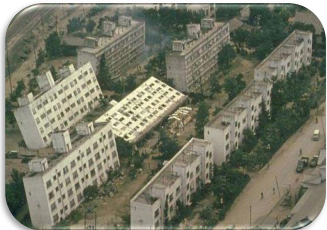
Liquefaction caused by the 1964 Niigata, Japan earthquake caused these apartment blocks to experience severe leaning. Image from the University of Washington.
