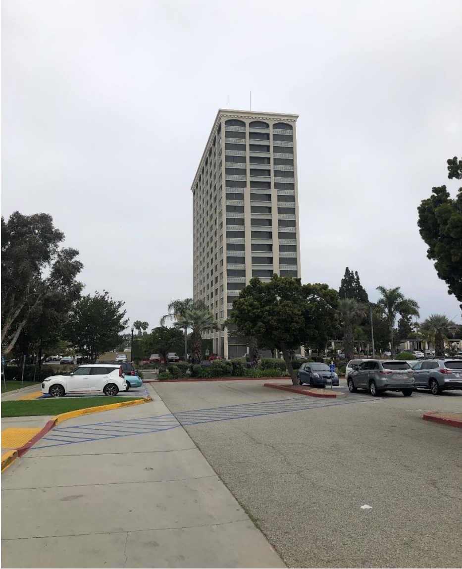
Existing affordable senior apartments (Tower on 19 th ), north of subject site
