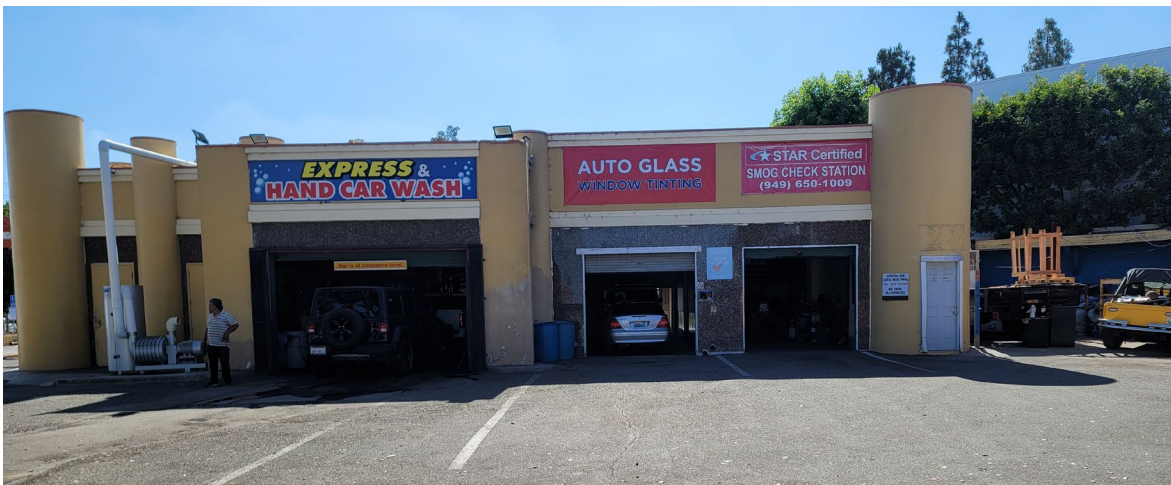
Image 1 – 2285 Newport Boulevard as Viewed Facing West
