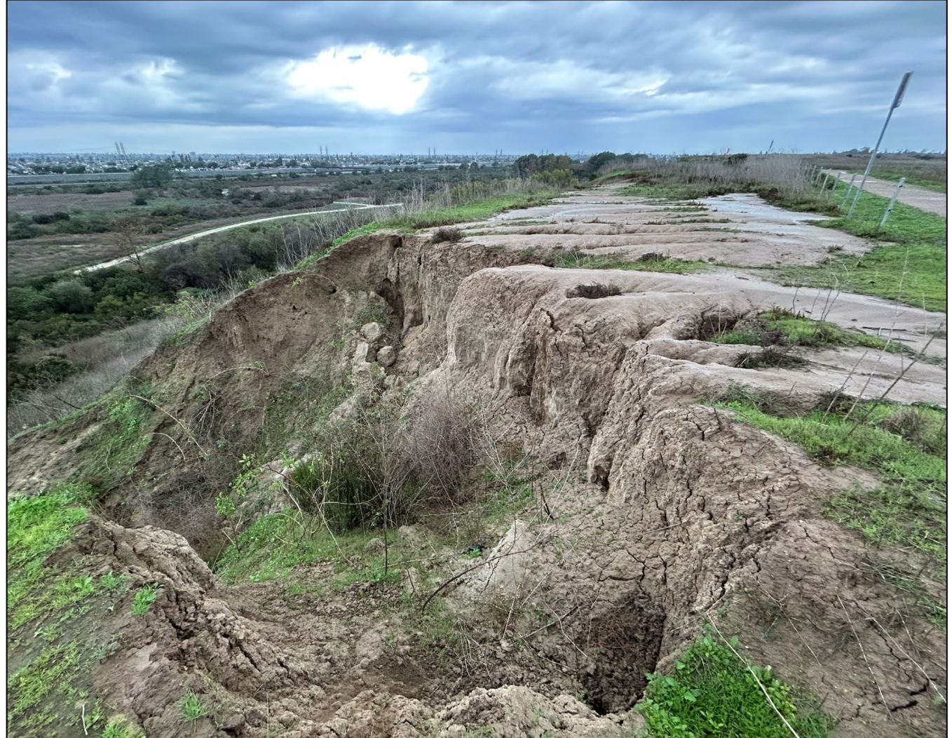
West Bluff Erosion
