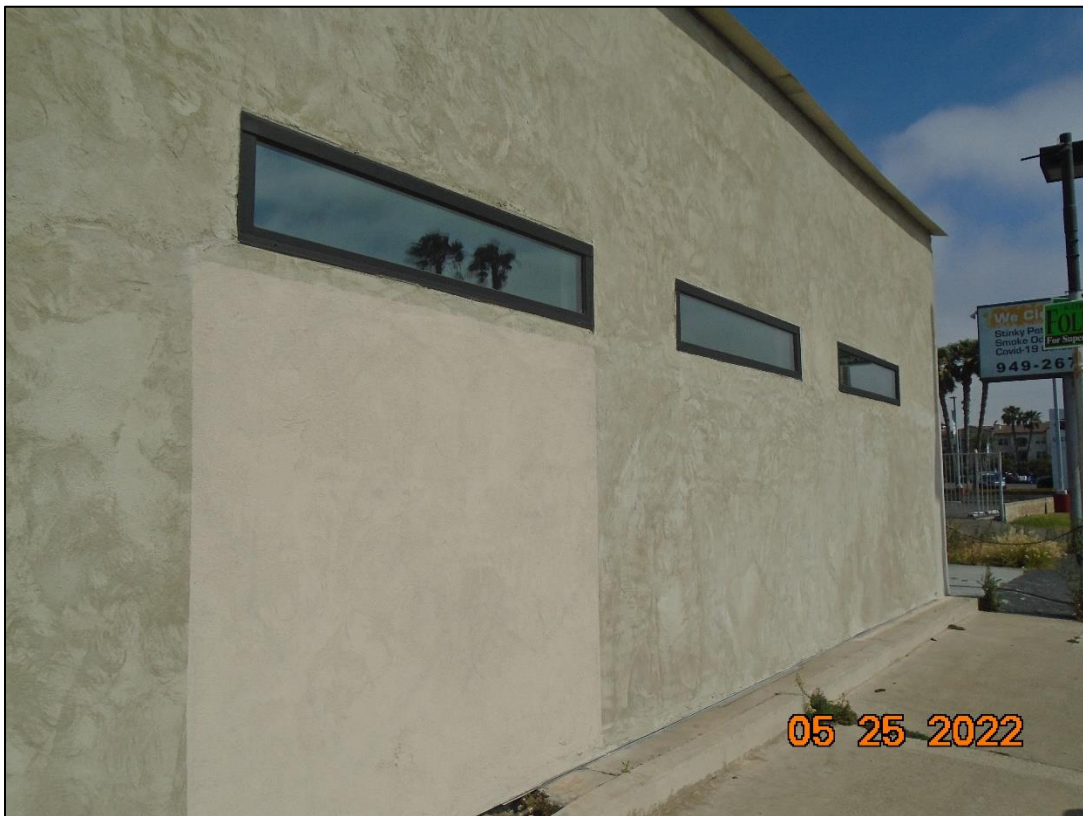
Façade remodel along Harbor Boulevard in progress
