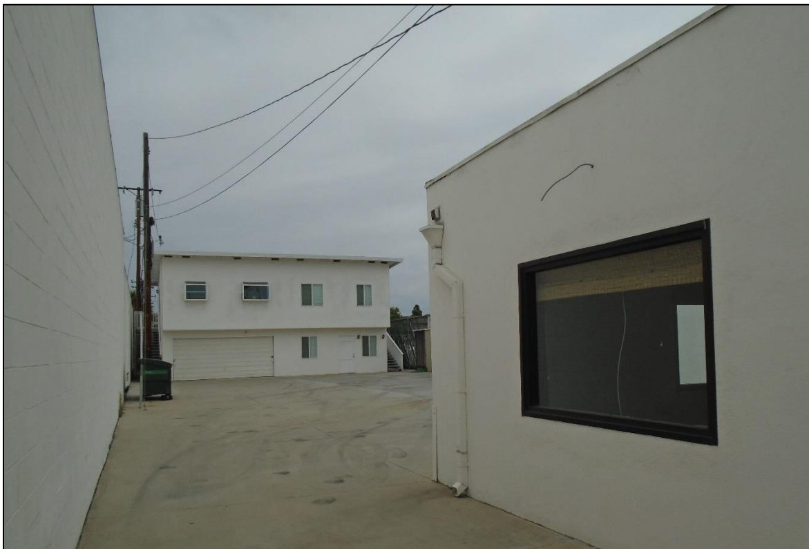
View of the rear front building and rear building
