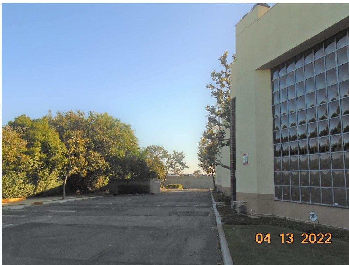
PA-22-01 Site Photos 3505 Cadillac Avenue, Unit O-102
