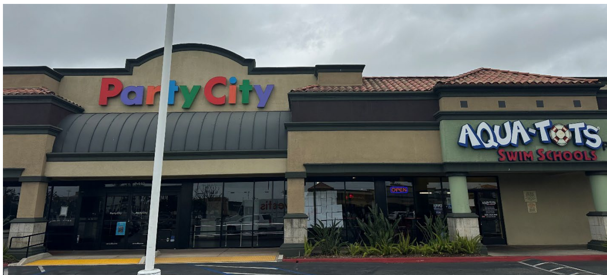
Figure 2. Existing Site Photo (tenant space)
