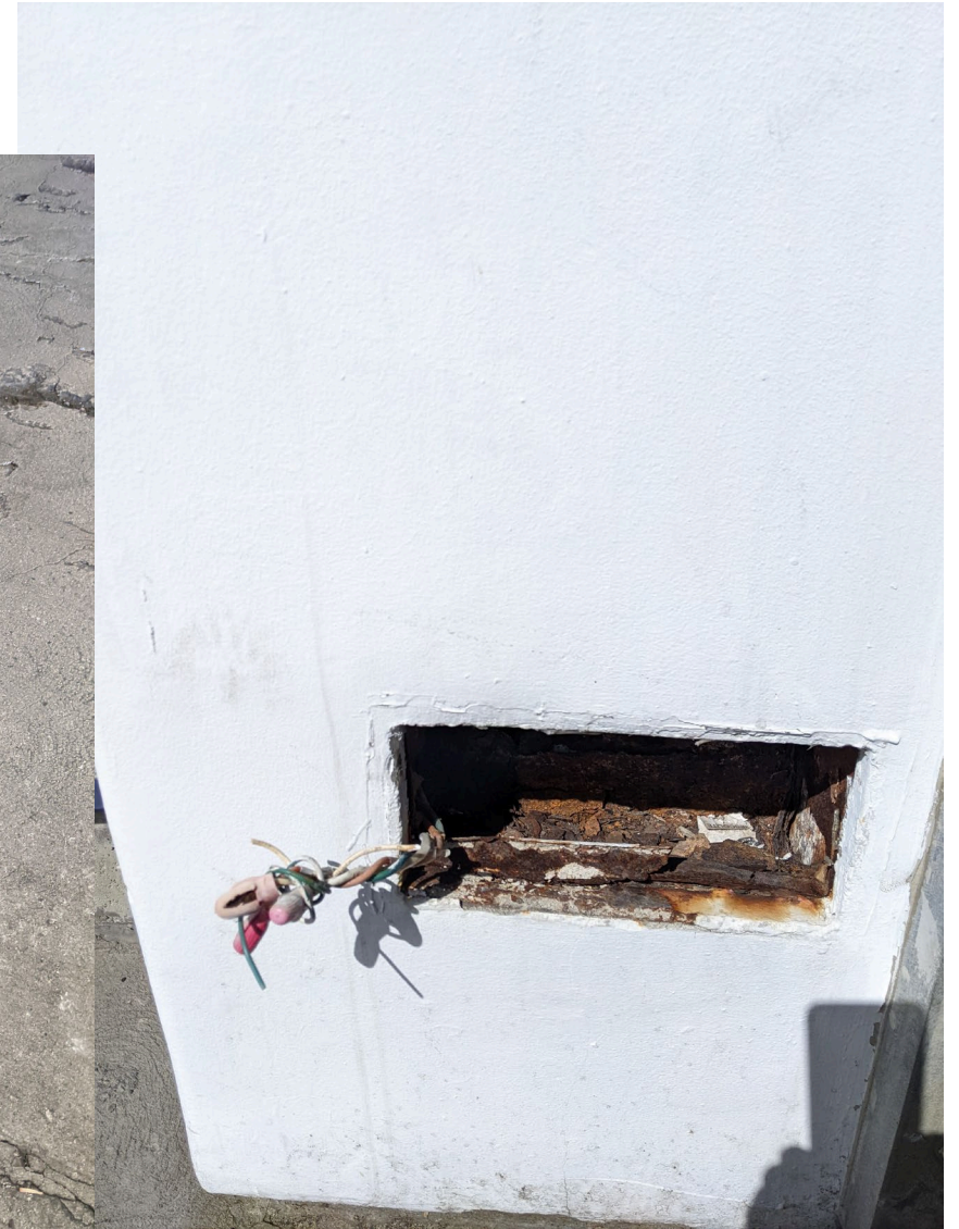
Broken Rusty Light
