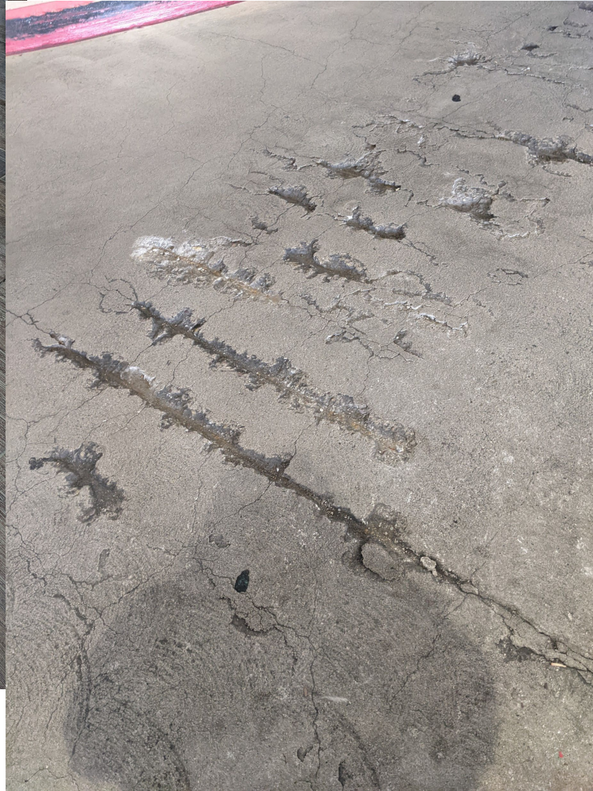
Exposed Rebar
