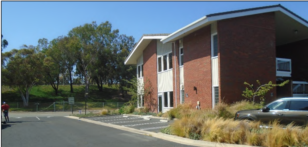
View of the side door (to become entrance) and parking
