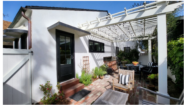
Figure 3. East elevation, view looking west. Source: GPA, February 2023.
