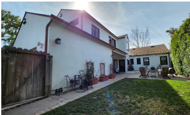
Figure 4: North elevation, view looking south. Source: GPA, February 2023.
