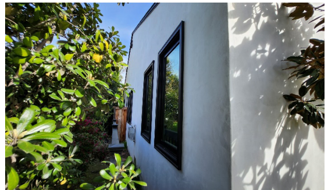
Figure 5: West elevation, view looking east. Source: GPA, February 2023.
